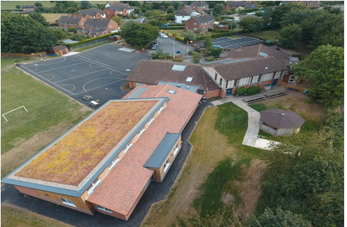
Leigh & Bransford Primary School - Extension
